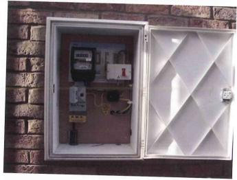
Please note that if your supply is being made with two separate cables then there should be two separate non-metallic cable ducts. Only NIE equipment should be located within an external meter cabinet, unless otherwise agreed with NIE. The bottom edge of the cubicle should be installed to be within 900mm to 1050mm from finished ground level.
